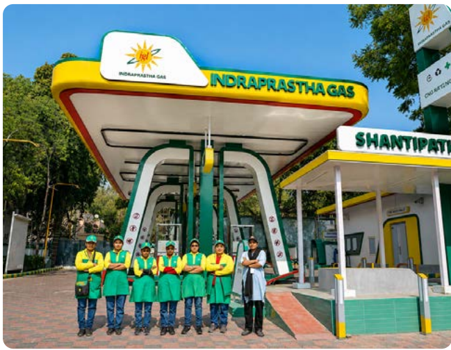
IGL upgraded Shantipath CNG COCO Station with Modern design & Modular structure
